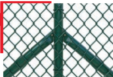
Brace Fixation Detail
