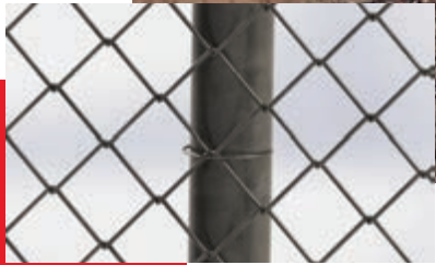
Tie Wire Fixation Detail
